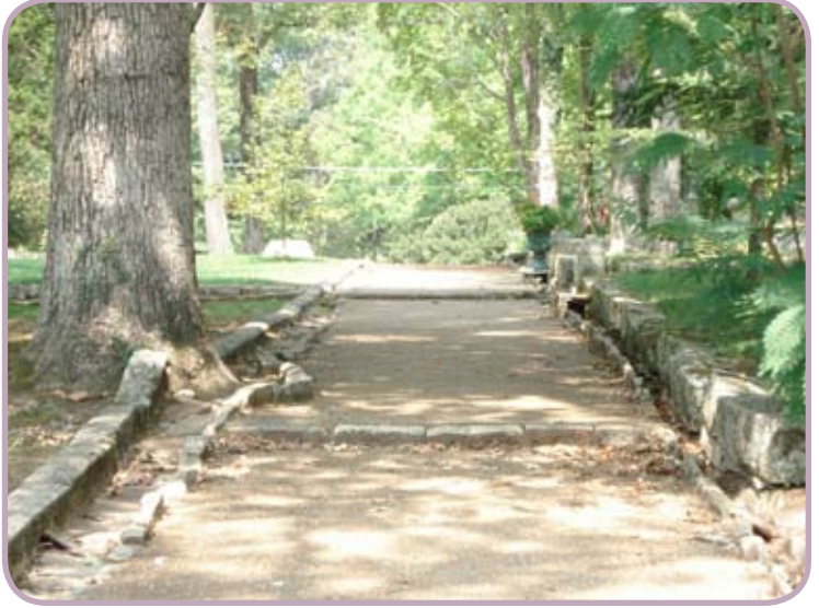
T4 - Gutter - Monteagle, TN
