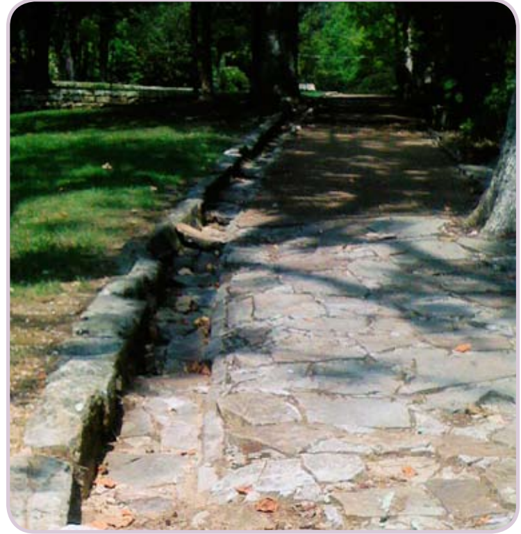
T3 - Gutter - Monteagle, TN
