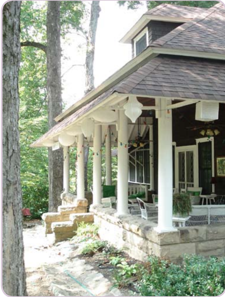
T3 - Gutter - Monteagle, TN
