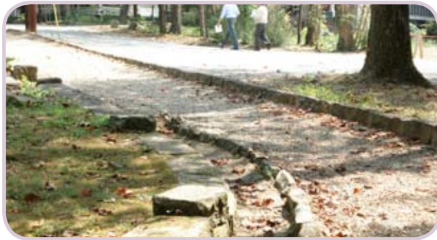
T3 - Gutter - Monteagle, TN
